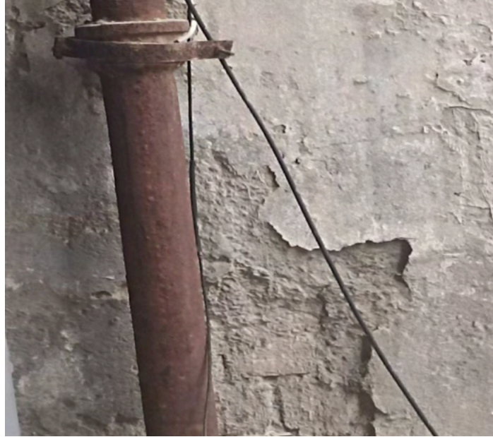
Image 5 & 6 : Showing mild decay of outer walls due to leakage at drainage pipes. (Image Credits : Author)
