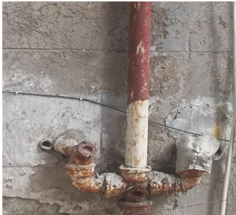
Image 4 : Showing mild damage to the outer wall at the water drainage system joint. (Image Credits : Author)
