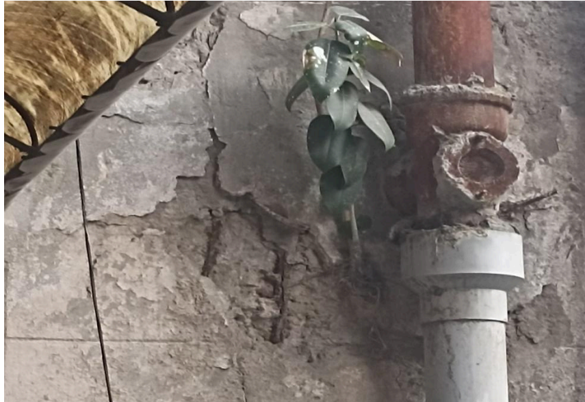
Image 4 : Showing mild damage to the outer wall at the water drainage system joint. (Image Credits : Author)
