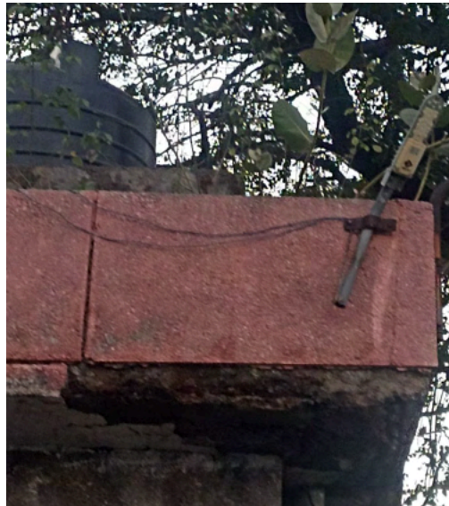
Image 7 : Showing moderate decay of slab due to overflow of water tank and improper drainage slope. (Image Credits : Author)
