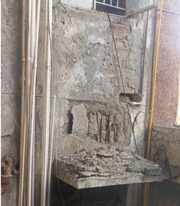
Image 10 : Showing severe decay outside of the kitchen wall near the water drainage system.
